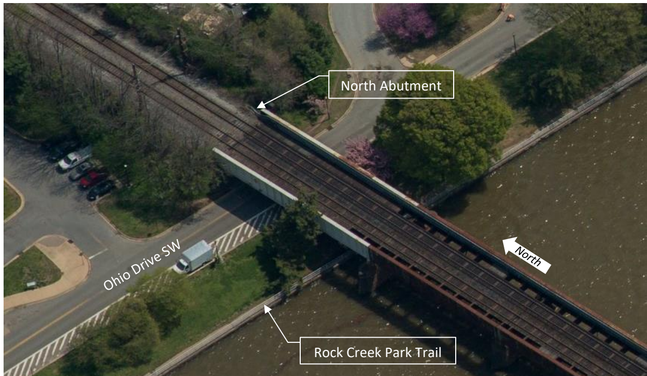
Figure 2-4 | North End over Ohio Drive SW and Rock Creek Park Trail
