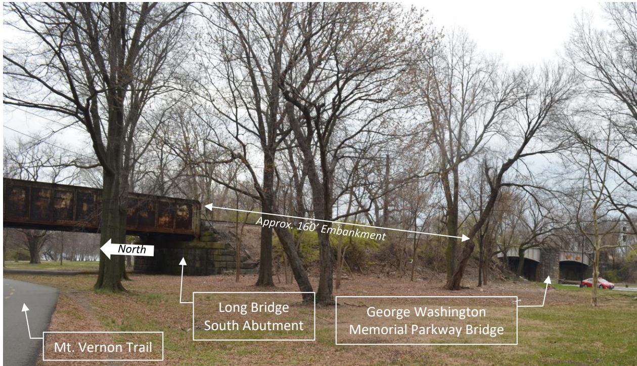
Figure 2-7 | Track Embankment beyond South Abutment
