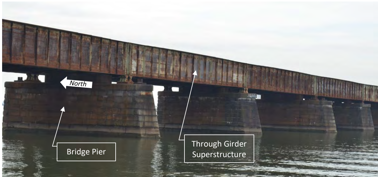
Figure 2-2 | Swing Span over Channel
