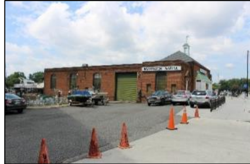
Figure 3-36 | Washington Marina Building
