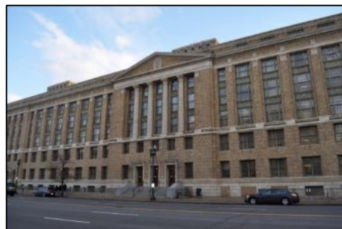
Figure 3-14 | USDA South Building
