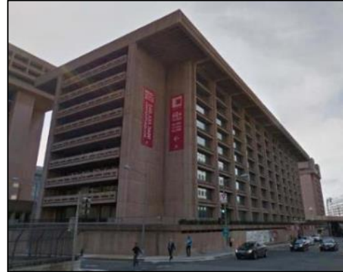
Figure 3-42 | Astral Building (Google Maps)
