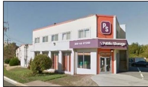
Figure 3-46 | 398 Long Bridge Drive (Google Maps)
