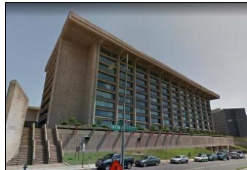
Figure 3-43 | Comsat Building (Google Maps)
