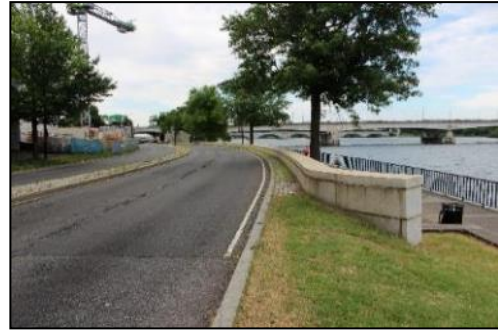
Figure 3-3 | Rock Creek and Potomac Parkway
