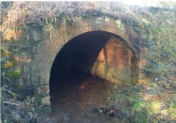
04-WTL-89-wet View of 7 foot, brick Culvert 04 feeding wetland from under railroad
