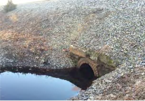
04-WTL-40-wet View of Culvert 02, concrete 36"
