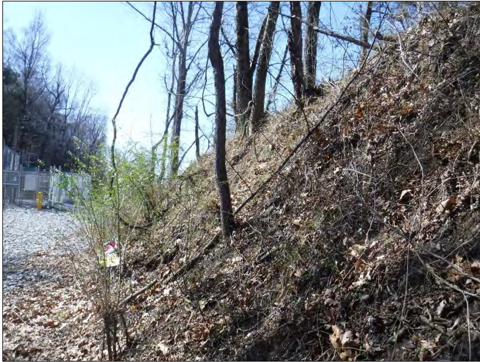
FIGURE 4-80: STEEP SLOPE IN AREA 3A, LOOKING SOUTH
