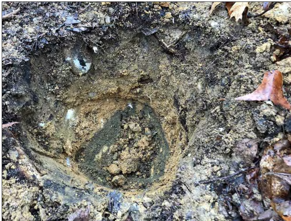
FIGURE 4-155: DISTURBED STP IN AREA 4F
