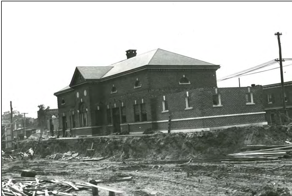
FIGURE 3-41: RENOVATIONS TO THE FREDERICKSBURG TRAIN STATION IN 1927 (HFFI 1927). NOTE THE LOWERING OF THE ROADWAY IN FRONT OF THE STATION.
