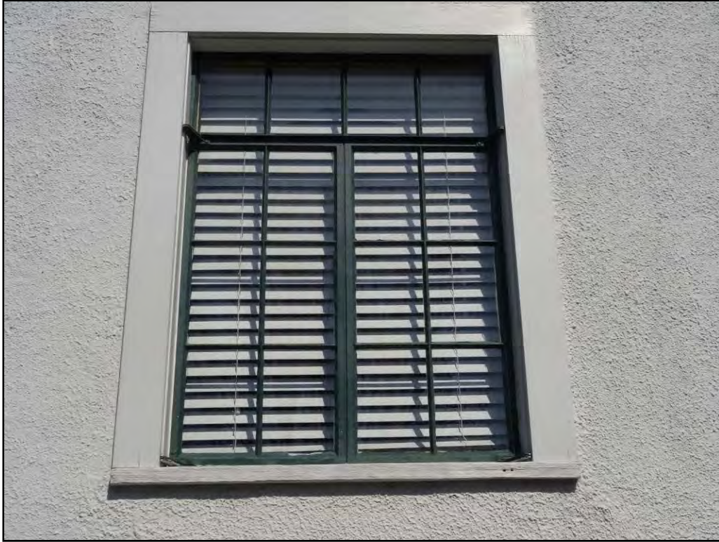
FIGURE 3-64: DETAIL VIEW OF METAL CASEMENT WINDOW
