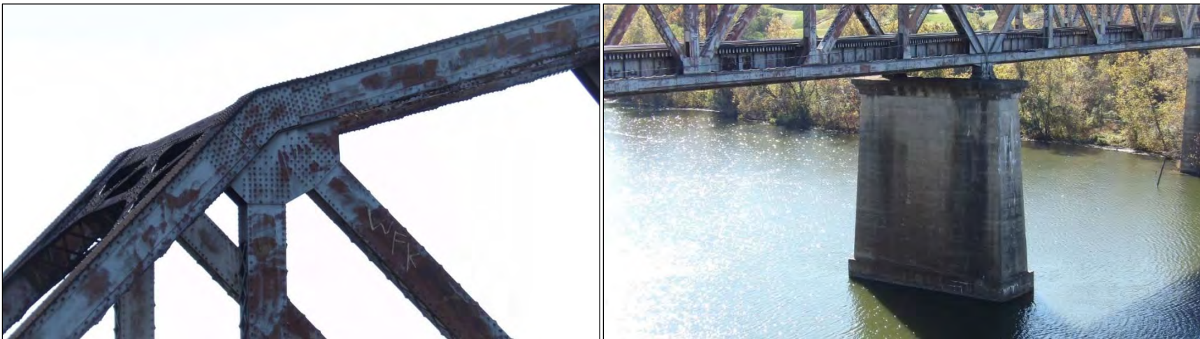
FIGURE 3-7: CLOSE-UP OF THE RIVETED CONNECTIONS ALONG THE TOP CHORDS AT THE NORTHERN APPROACH (LEFT); CLOSE-UP OF ONE OF THE POURED CONCRETE SOLID-WALL PIERS, LOOKING SOUTHEAST (RIGHT)
