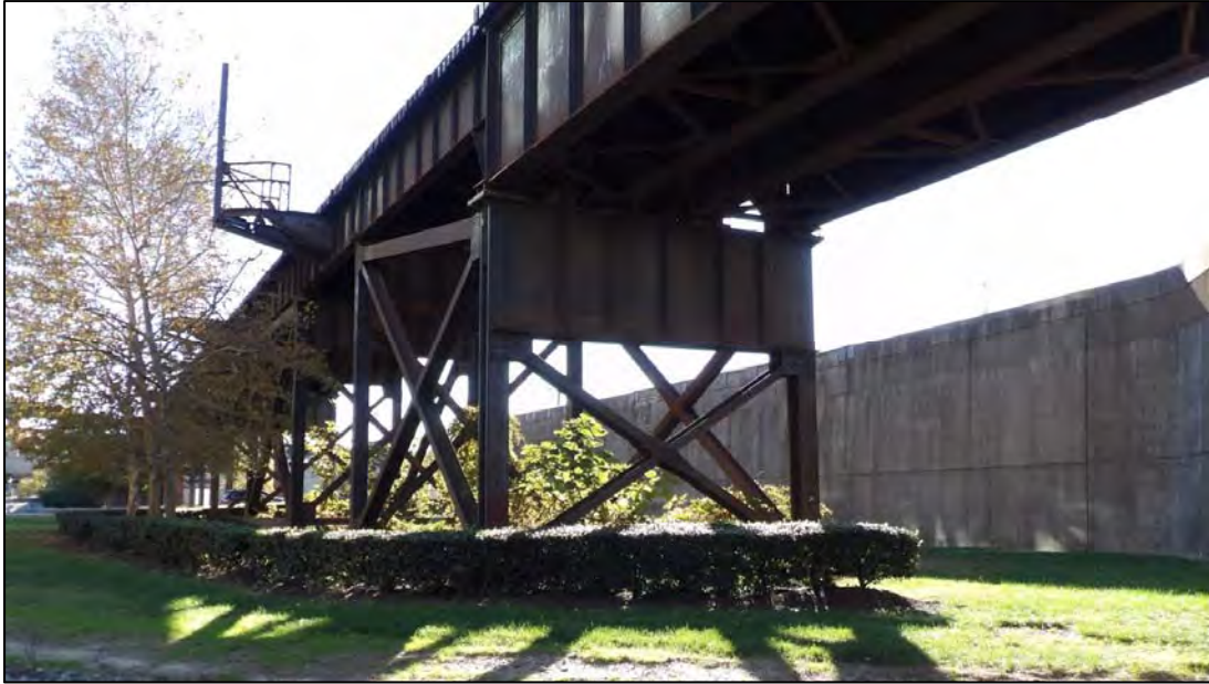
FIGURE 3-148: A C&O ELEVATED STEEL-PLATE-GIRDER BRIDGE AT SOUTH 14TH STREET, RICHMOND, VA, LOOKING SOUTHWEST
