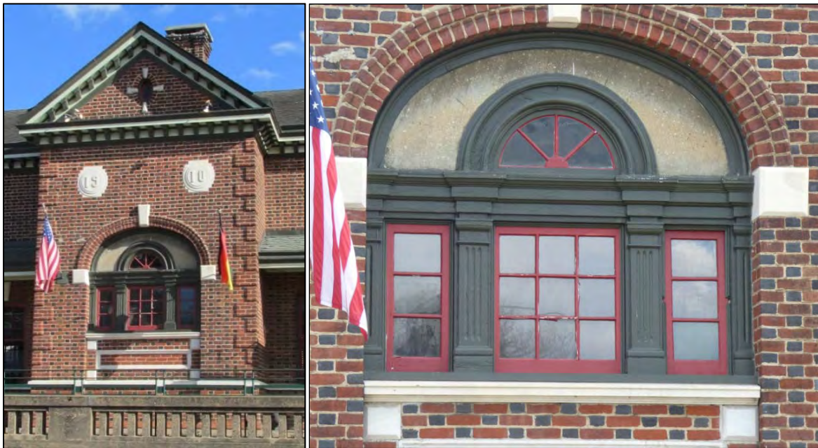
FIGURE 3-47: FREDERICKSBURG TRAIN STATION, DETAIL OF PROJECTING BAY AND PALLADIAN WINDOW ON NORTH ELEVATION
