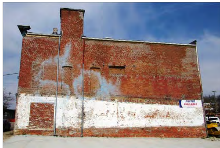
FIGURE 3-207: GHOSTING ON SOUTHWEST ELEVATION
