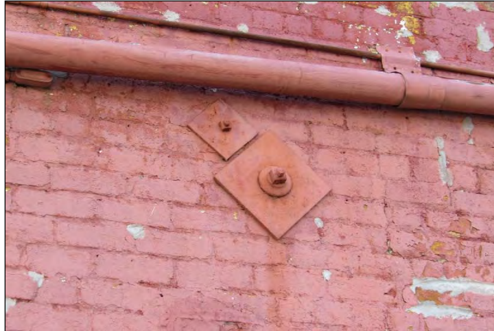
FIGURE 3-205: ANCHOR PLATE AND TIE ROD DETAIL
