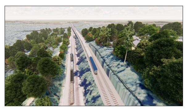
Figure 3: Original Rail Alignment (Left) and Proposed Elevated Bypass (Right) in the Northern Section of the Franconia Third Track Section, Looking South.
