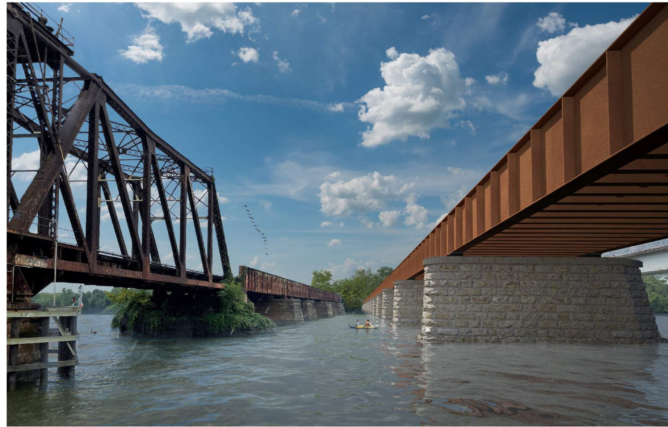
POTOMAC RIVER RAIL BRIDGE OVER POTOMAC RIVER (1) (LOOKING WEST)
