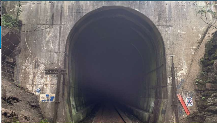
Slate Hill Tunnel
