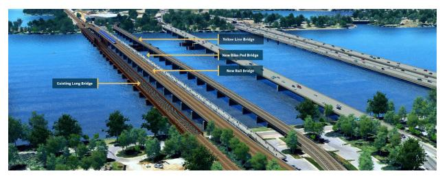
A rendering of the Long Bridge Project section over the Potomac River highlighting the new rail bridge and new bicycle-pedestrian bridge.
