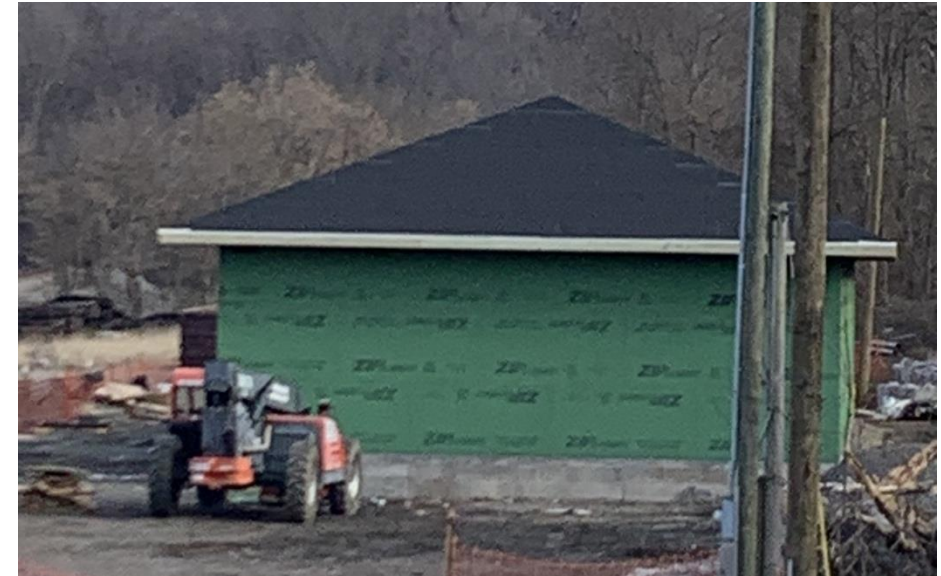
New NS Maintenance of Way Building (12/26/24)
