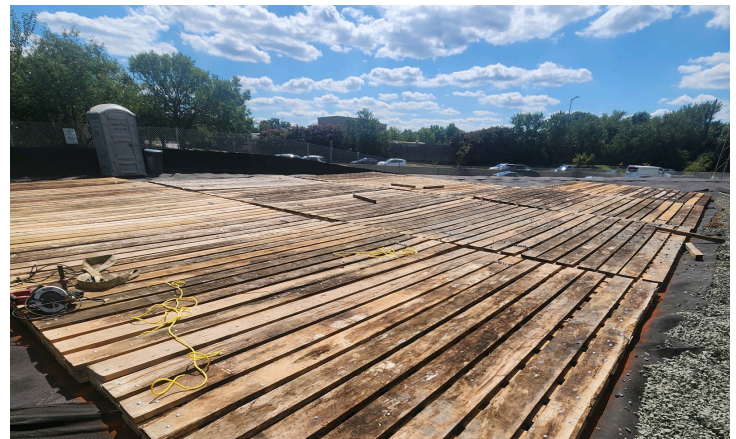
Designated protected areas will be shielded with root protection matting and fencing; stone or crane mats will be used for additional protection as needed.
