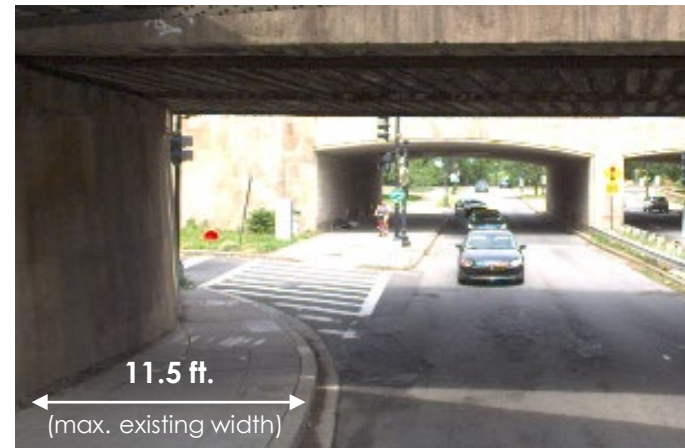
Existing Trail/Sidewalk Width under Existing Rail Bridge
