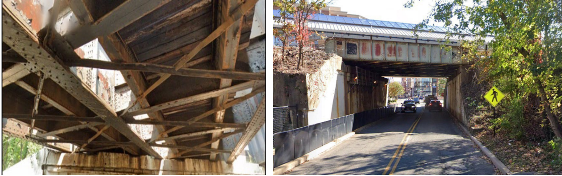
Existing King Street Rail Bridge
