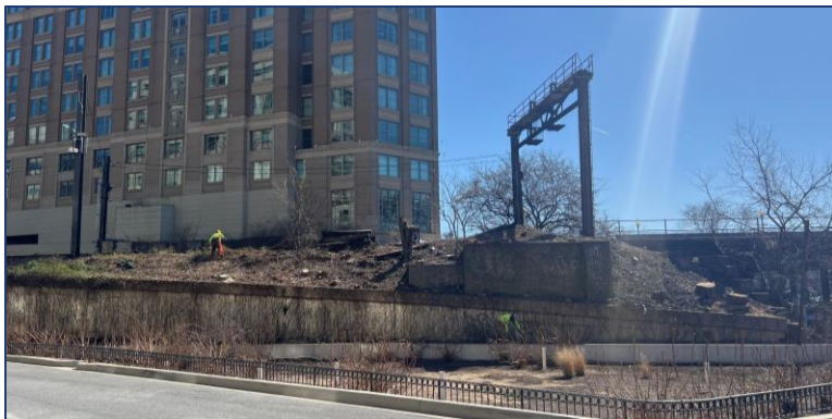
Select tree removal is happening along the Long Bridge North corridor.
