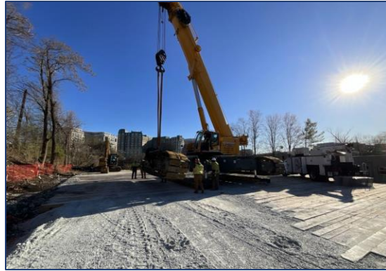
Site prep and crane assembly have been completed ahead of work on demonstration drilled shafts and micropiles in East Potomac Park, DC. These elements will better inform final design.
