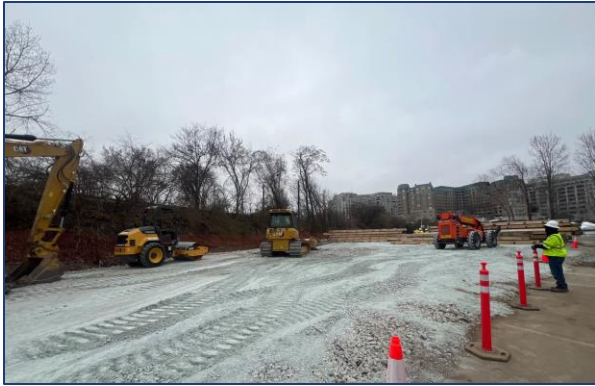
Site prep and crane assembly have been completed ahead of work on demonstration drilled shafts and micropiles in East Potomac Park, DC. These elements will better inform final design.
