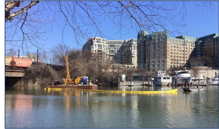
Geotechnical drilling work is underway in Washington Channel.
