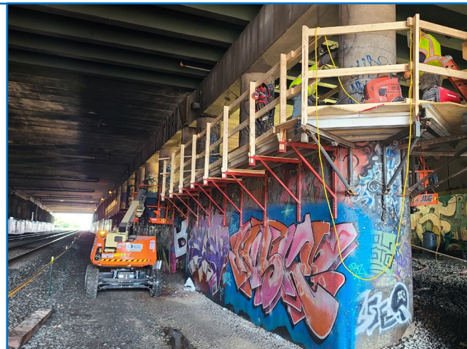
Following completion of track removal under Maryland Ave, crash wall strengthening work is underway.
