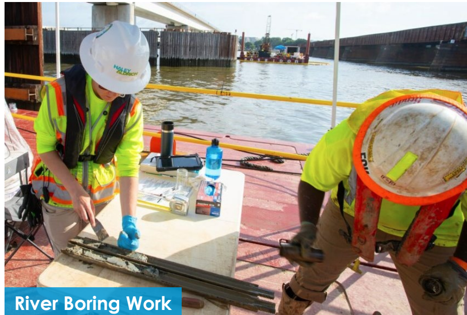
River Boring Work
