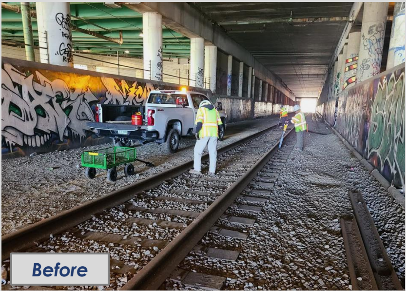
Out-of-service track was removed in May to enable construction on the crash walls.
