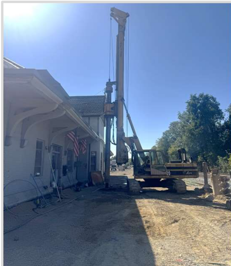
Drilled pier foundations for passenger platform and canopy
