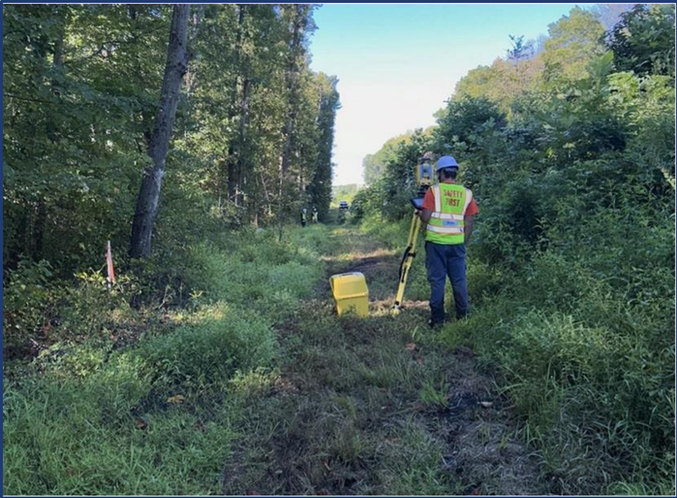
Contractor performing clearing, grubbing, preconstruction survey, and locating underground utilities.
