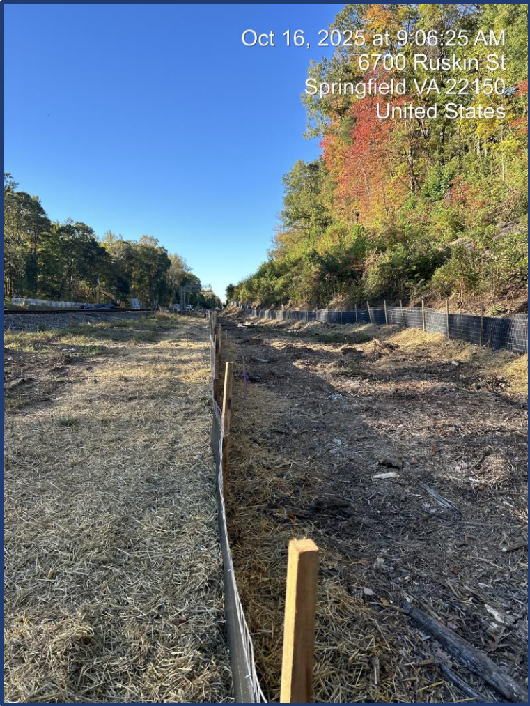
Erosion and sediment controls along the east side of the tracks
