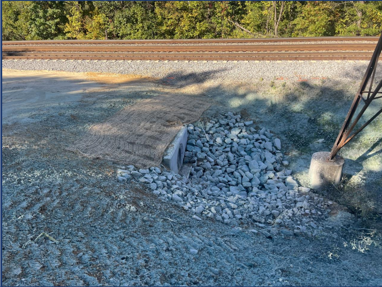
New stone and erosion control materials added around a drainage pipe to help stabilize area near new CP Beltway.
