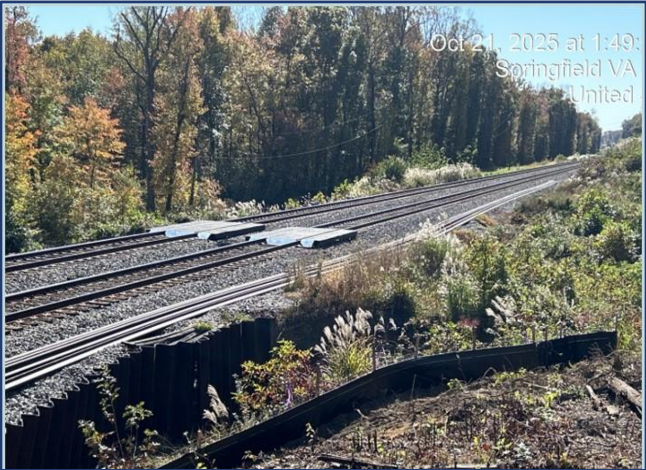
One of three track crossings installed by CSX to allow for more efficient contractor movements between west and east side of the tracks
