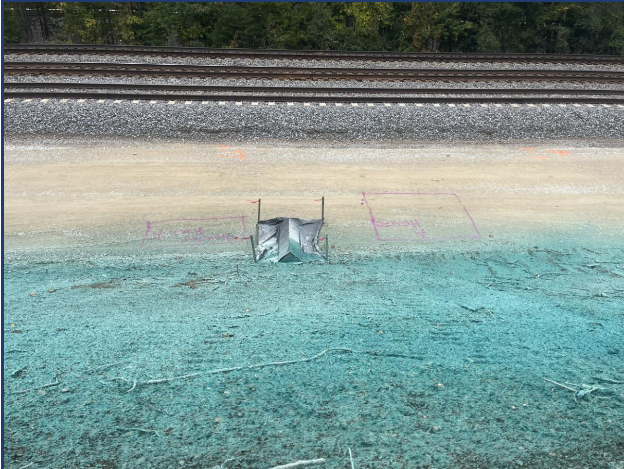
Crews marked out location of new signal equipment at new CP Beltway. Nearby slope was seeded to prevent erosion.
